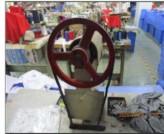
Photo of non-conformity NC The buttoning machine was not installed with pulley protection cover.JPG
