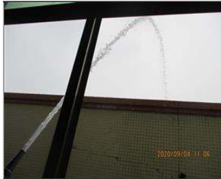
Photo of fire safety equipment Hydrant test.JPG
