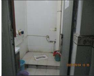
Photo of the sanitary facilities Toilet.JPG
